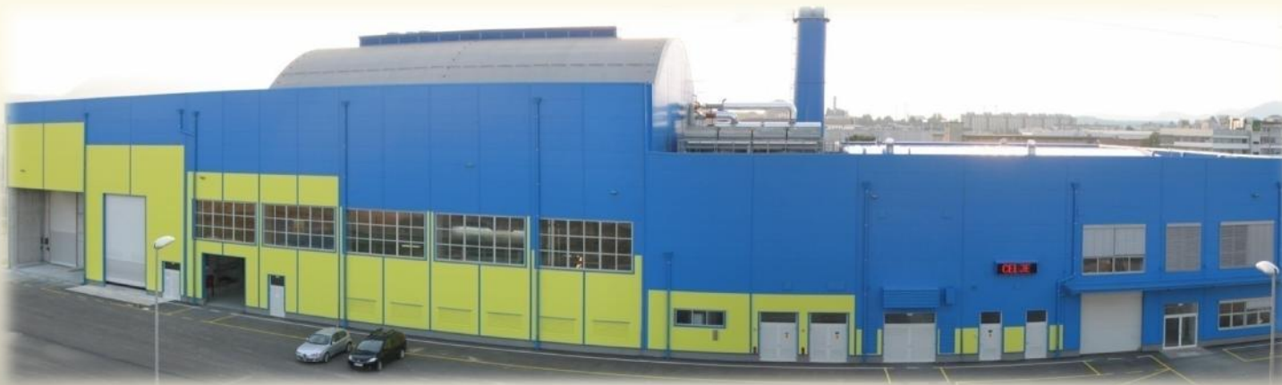
Celje W t E CHP Plant
